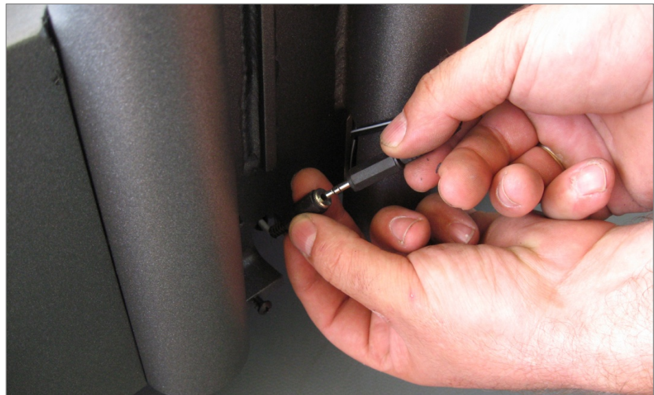
Fig. 14 Installation step, connect wires (CURVE / CURVE XL)
