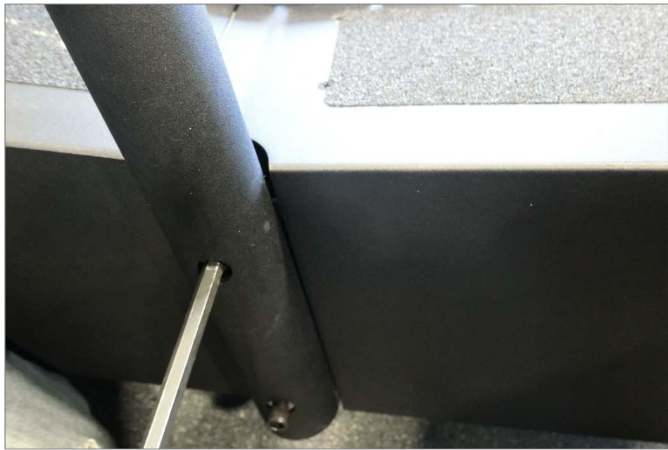
Fig. 20 Installation step, fixing the railing (CURVE TRAINER)
